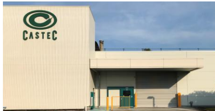
CASTEC inc. Head Office and Plant-1
