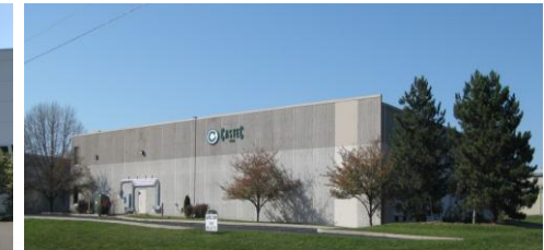
CASTEC corp. Office and Plant
